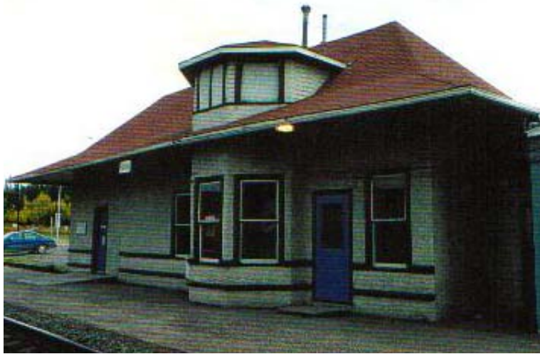
Original Location along CN mainline
